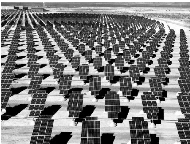
Figure 11.14. The largest photovoltaic solar power plant in the United States is at Nellis Air Force Base with the size of 70,000 solar panels worth 15 mega watt of power. Using about 140 acres of unused land. Courtesy of the U.S. Air Force, Neils Air Base.
